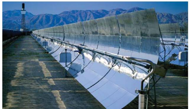
Solar-thermal parabolic trough power plant
